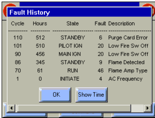
Fig. 62. Burner Control—fault history.
