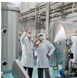
Pharmaceutical water treatment
